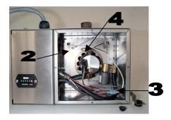
5. Remove igniter. Examine for damage/wear. Replace if necessary.
